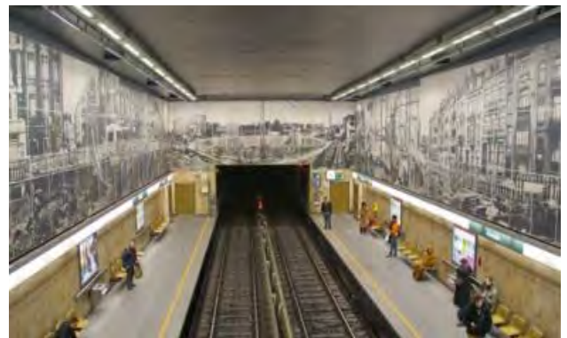
LED lighting upgrade at a station in Brussels, Belgium has reduced energy consumption by half Source: http://www.schreder.com
