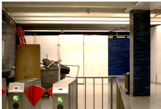
Figure 20: Maintenance Equipment Stored in Public View
